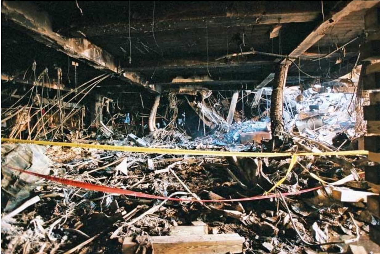
In this photo we see a massive amount of debris at the ground floor level. The plane would have passed diagonally from right to left across this scene and we observe that the support columns all appear to have been pushed to the left, as would be expected. In some cases only the reinforcing rods remain.
